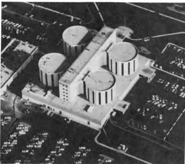
1982 All four towers completed. Mission accomplished!
