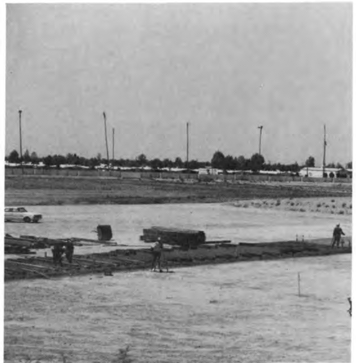
August 5, 1969 Construction gets underway.
