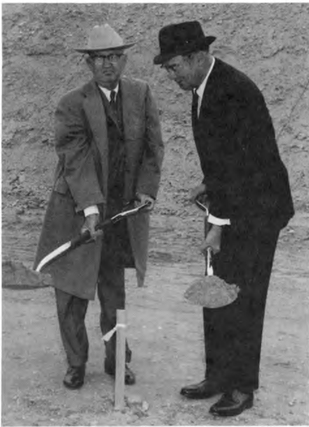
January 24, 1969 Groundbreaking (L to R) William W. Boswell, Brother of W.O. Boswell Del Webb, President, Del Webb Corporation
