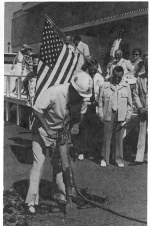
July 19, 1976 Third Tower groundbreaking.
