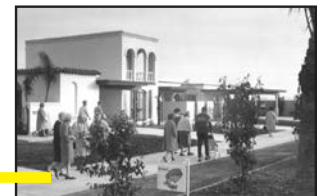
1968 Spanish and Mediterranean villas introduced at 105th Drive, west of Mountain View. There was an all-electric experimental home at 9746 N. 105th Ave.
