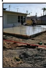
May 17 Foundation poured.
