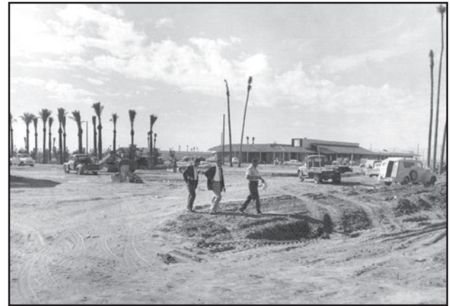
Entrance to Sun City under construction. Dec. 4, 1959.
