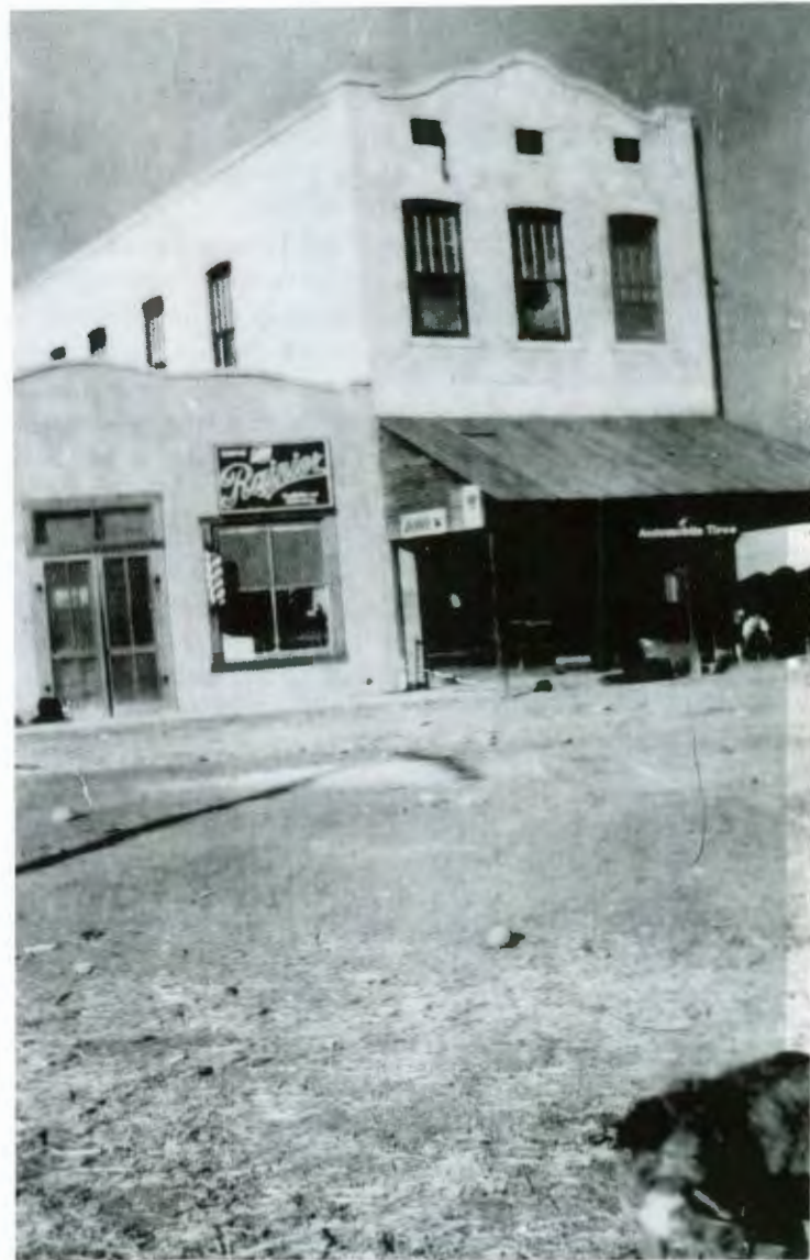
Marinette’s General Store once stood near the present-day intersection of 105th Avenue and West Thunderbird Boulevard.
