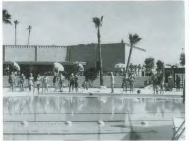
Town Hall South Recreation Center and pool.
