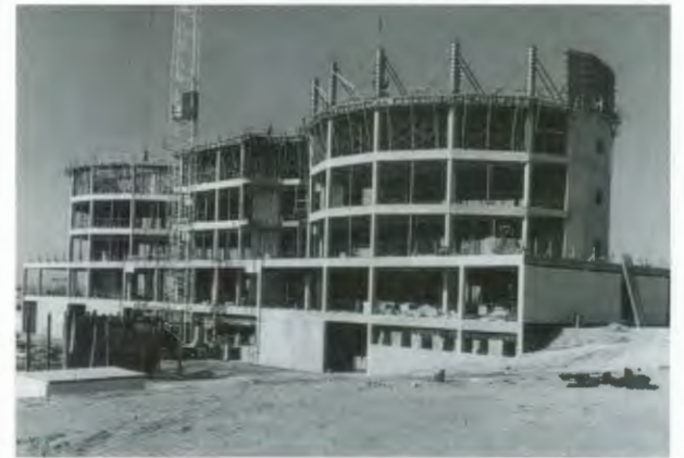
Walter O. Boswell Memorial Hospital under construction.
