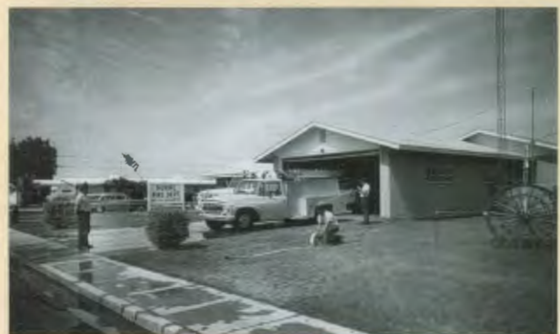
Top: The Lakes Club, the community's largest private country club, is destroyed by fire one month before opening, but reopens seven months later. Above: Sun City's first fire station, at 111th and Grand avenues, was equipped with a single pumper truck.
