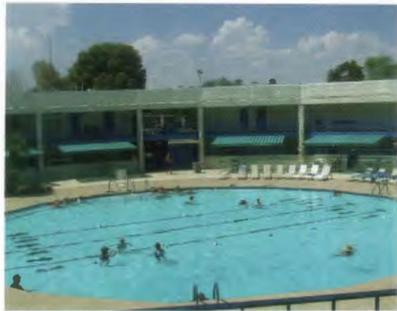
The Lakeview Recreation Center swimming pool.
