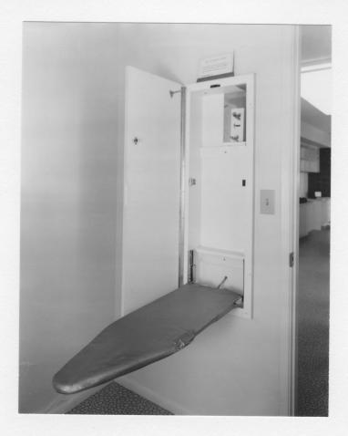
A built-in ironing board made by Iron-A-Way was installed in the utility room specifically to determine its desirability for our market. This unit was recessed into the wall between two studs. The case was made of wood and had a door. The exposed door and sides of the case were painted the wall color resulting in a neat, unobtrusive arrangement. The board, which had a 4-inch adjustment up or down, was three feet long. There is
