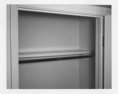
Three different types of wardrobe closet shelving were used in this house. One of these was the conventional wood shelving with a clothes pole which we have been using for years. The second type was a 3/16" diameter, plastic-coated wire-rack type manufactured by Pemco.
