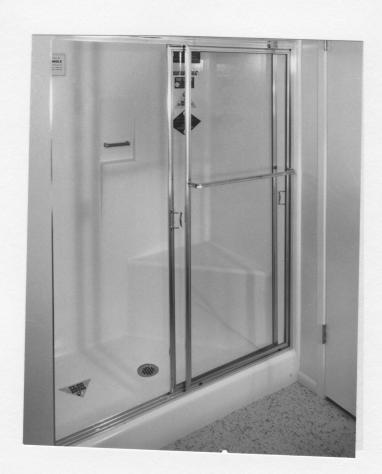
Bathing fixtures made of fiberglass, manufactured by the Universal-Rundle Company, were installed in the baths. These bathing fixtures have been improved substantially during the last year and a half owing to improved unit design, production techniques, quality control procedures and improved gel-coat materials. (See HS-2, January 6, 1965). These fixtures were white with gold fleck. The same fixtures are available in the standard Universal-Rundle fix-
