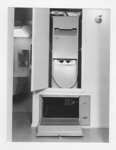
Noise from the gas furnace blower and combustion has long been a source of customer complaint. An attempt was made here to solve this problem and it was highly successful. Two principal steps were taken here:
