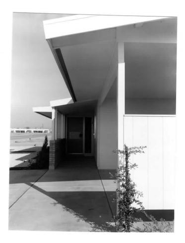
A soffited overhang was included in this house in order to compare its appearance with that of houses nearby having exposed rafter tails, and to gain first-hand experience with costs toward the end of eliminating those callbacks common to exposed overhangs. Regular half-inch gypsum board was used for the soffit material owing to the dryness of the area. There is no concern about using interior gypsum wallboard for this application. It has been used here
