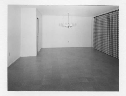
Corkwood is a block flooring 3/8" thick and 9" square, tongue and groove with a grooved back. It is made from grated wood chips impregnated with synthetic resin, formed and cured under heat and pressure. It is said to resist indentation 2 1/2 times as well as oak. It may be installed over wood or concrete. It is set in a mastic. It is available in two colors, light and dark.
