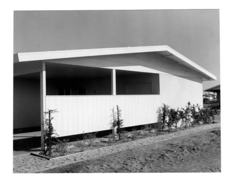
This fence is framed with 2 x 4's having 4'-0" panels of Ruf-X-Ninety masonite hardboard nailed to its exterior side. It has a redwood cap.
