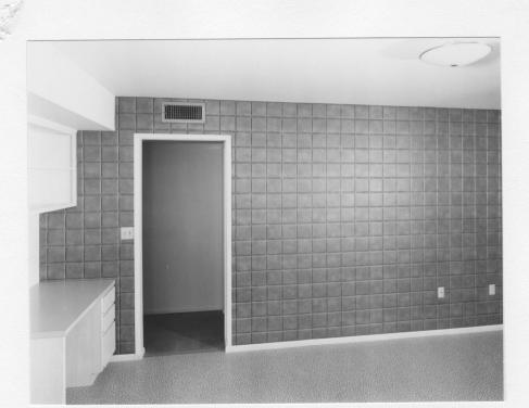
This vinyl wall covering made by Colamco is distinctive for its deep relief in the pattern. The exposed vinyl has a 3/8" thick urethane blanket backing which is covered by muslin. The patterns are almost unlimited. They are made by the use of ribbon dyes and heat. The material is made in 4'-0" x 8'-0" sheets. The colors and textures of the vinyls offered are also almost unlimited. The material is hung on the wall by the use of a synthetic adhesive used for hanging wall paper.
