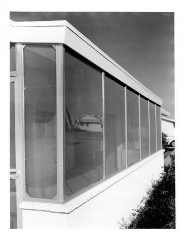
The lanai enclosure framing members were made of architectural aluminum extrusions now in common use for this purpose, and Fiberglass screening. This section of the enclosure was set on a 30" high, 6" concrete block wall having an 8" wide cap. The 8" cap was used for appearance sake but it turned out to be a mistake in that it just catches rainwater dripping from the roof. It should have been a 6" cap. The enclosure has a quality door.
