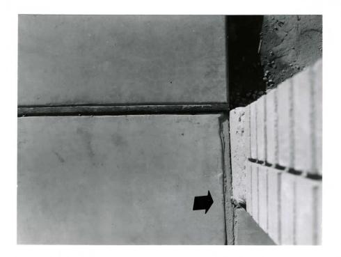
Homasote expansion joint called Homex was installed at the joint between the front porch floor and the driveway. This material is made of wood fibers derived from the repulping of No. 1 grade news stock with waterproofing ingredients added. It is available in the standard sizes that all other expansion joint materials are available in. Homex expansion joint meets federal specification, HH-F-341a and American Association of State Highway Officials Specification M-153-54, Class III.
