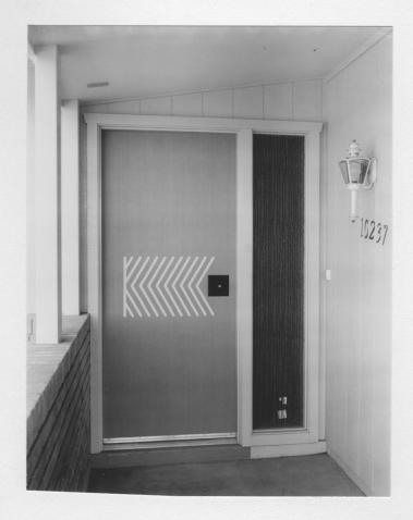
The distinguishing feature of the front entry door in this house is that the exterior skin, which is made of tempered hardboard, has a burlap-like texture with a contemporary design milled into it.
