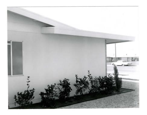
A material called Tex-Cote, manufactured by Textured Coatings of America, Inc. in Los Angeles, California, was selected from several others to be used on the exterior walls of this Research House. Tex-Cote was developed during World War II when it became imperative to have coatings which would protect military equipment in all climatic extremes. Subsequently, it has been
