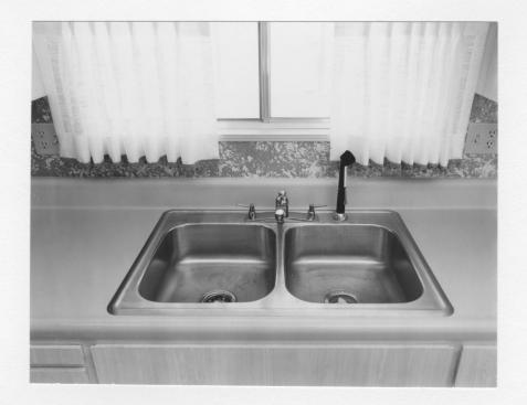
The kitchen sink was a seamless, double compartment Elkay sink, Model 43322, drawn of No. 20 gauge non-nickel bearing, type 430, stainless steel. All exposed surfaces have a No. 4 satin grind finish. The interior corners of the compartments have a minimum 3" radii. A sound dampening material is applied to the underside of the sink. The mounting rim is integral with the sink (separate mounting frame not required).
