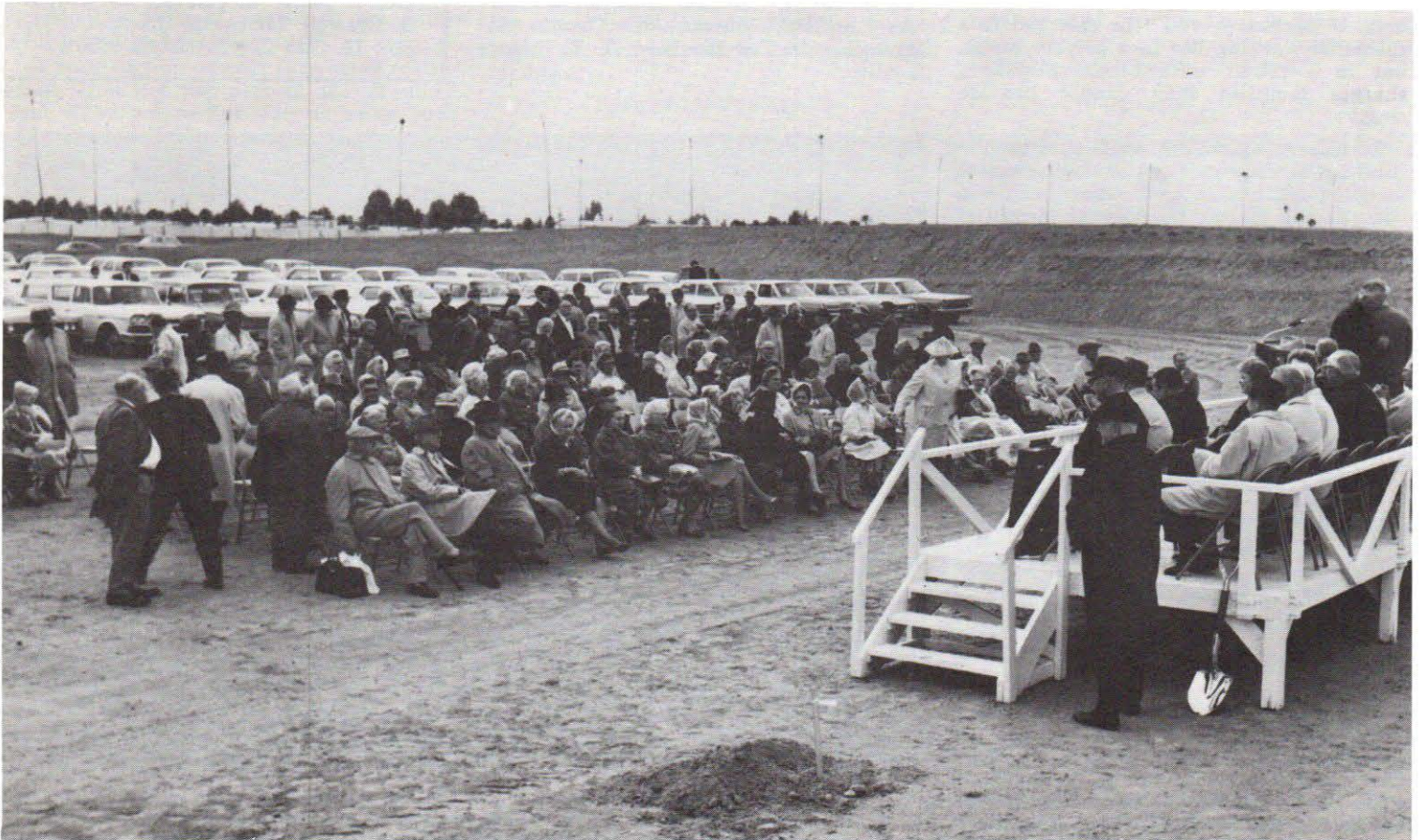
Despite chilly weather, an estimated 300 persons attended the groundbreaking ceremonies on Thunderbird Road between 103rd and 105th Avenues. Some of those standing are not shown.
