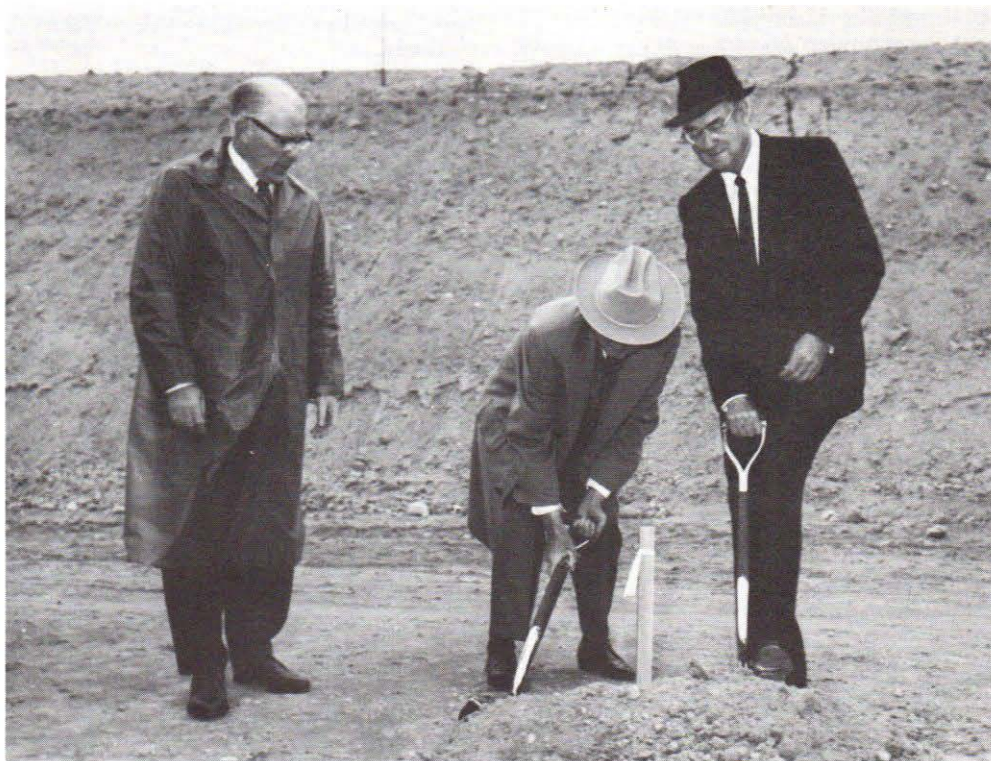
William W. Boswell (left) and Del E. Webb turned the first shovelful of earth at the Jan. 24 groundbreaking ceremonies for the Walter O. Boswell Memorial Hospital in Sun City. At Boswell's left is W. A. Chapman, president of the Sun City Community Hospital, Inc., the hospital corporation. The top of the bank in the background will be approximately the ground floor level of the hospital.
