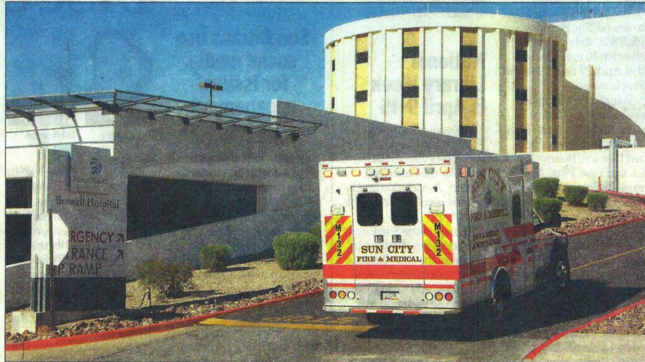
Banner Health officials are preparing for additional design development for a reconfiguration of the Boswell Medical Center emergency department to eliminate the ramp to the entrance. [Independent Newsmedia/Rusty Bradshaw]
