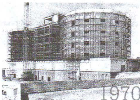
Boswell Hospital's first two towers are under construction and set to open in November.
