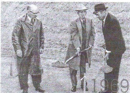
William Boswell (center) lifts the first shovel of dirt at the 1969 ground-breaking ceremony. William Chapman of DEVCO is to his right, and Del Webb is to his left.
