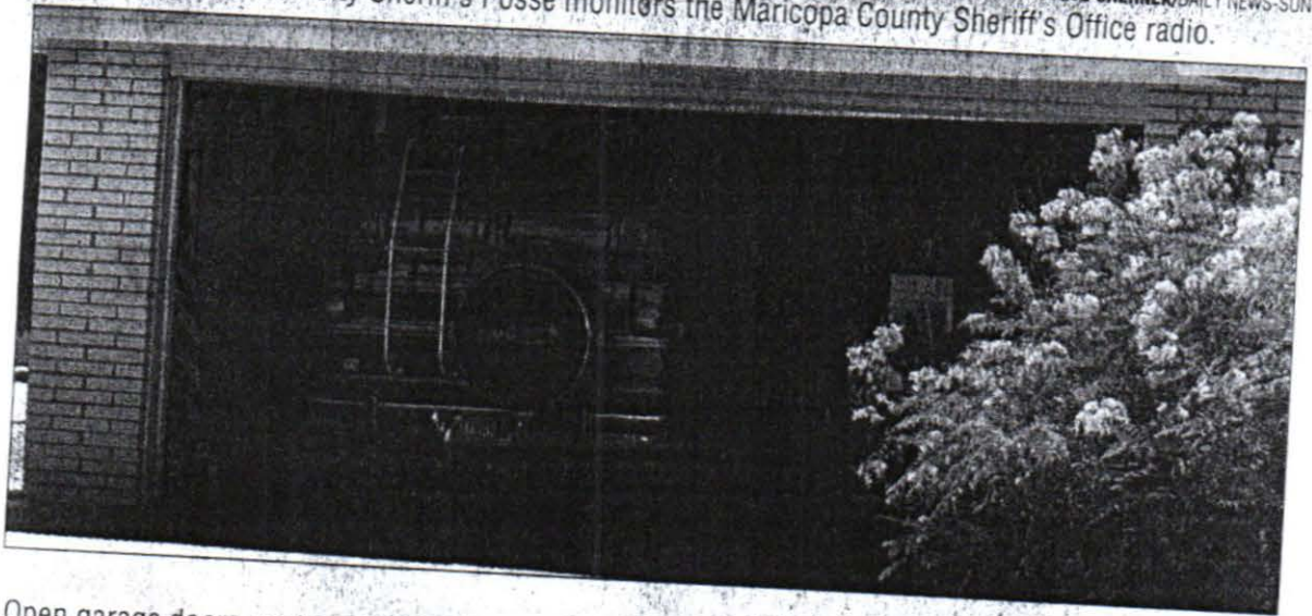
Open garage doors are tempting for would-be thieves and contribute to crimes of opportunity. STEVE CHERNEK/DAILY NEWS-SUN
