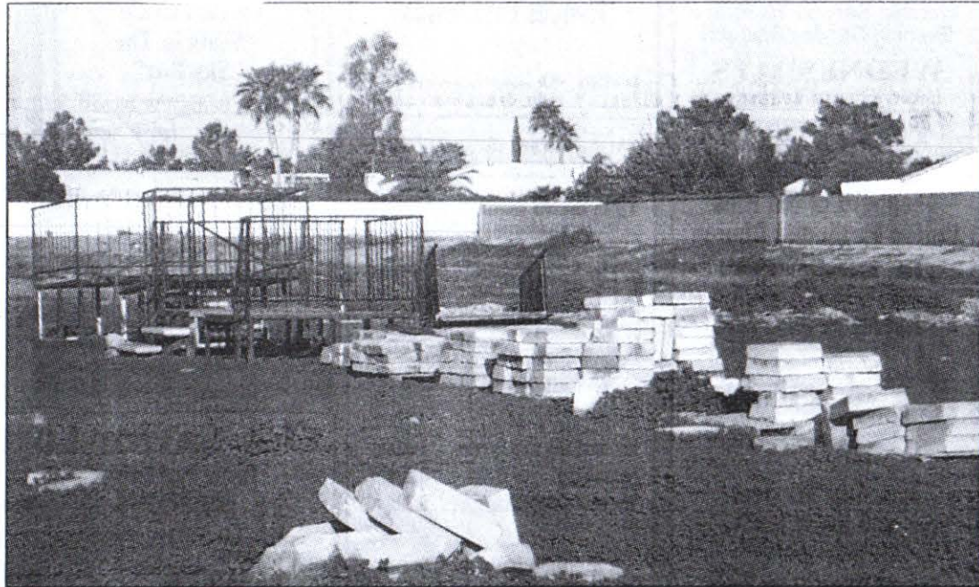
From the northeast corner of the proposed transportation yard, both the Sun City, left, and Brookside Village property walls are visible.
