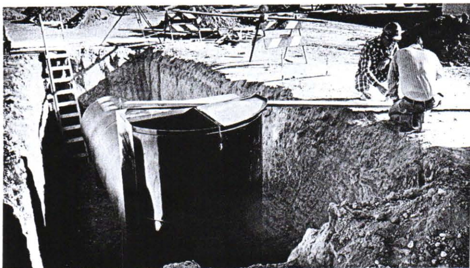
The 2,000-gallon tank that is stored beneath the ground to function within the solar system.
