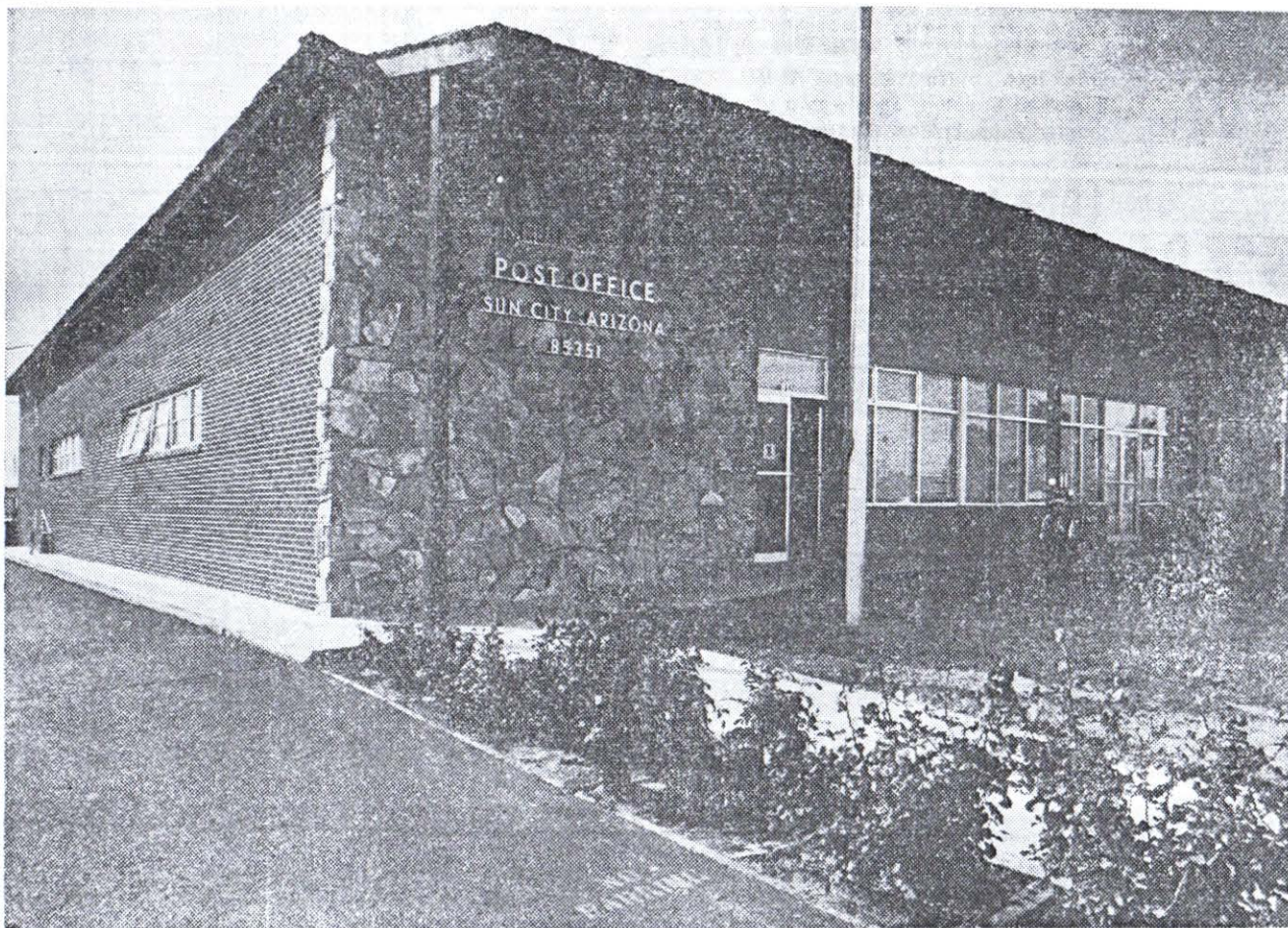
Exterior of Sun City's old Post Office at 103rd Avenue and Coggins Drive.
