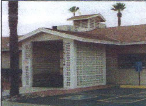
Front Entrance to Oakmont early on
