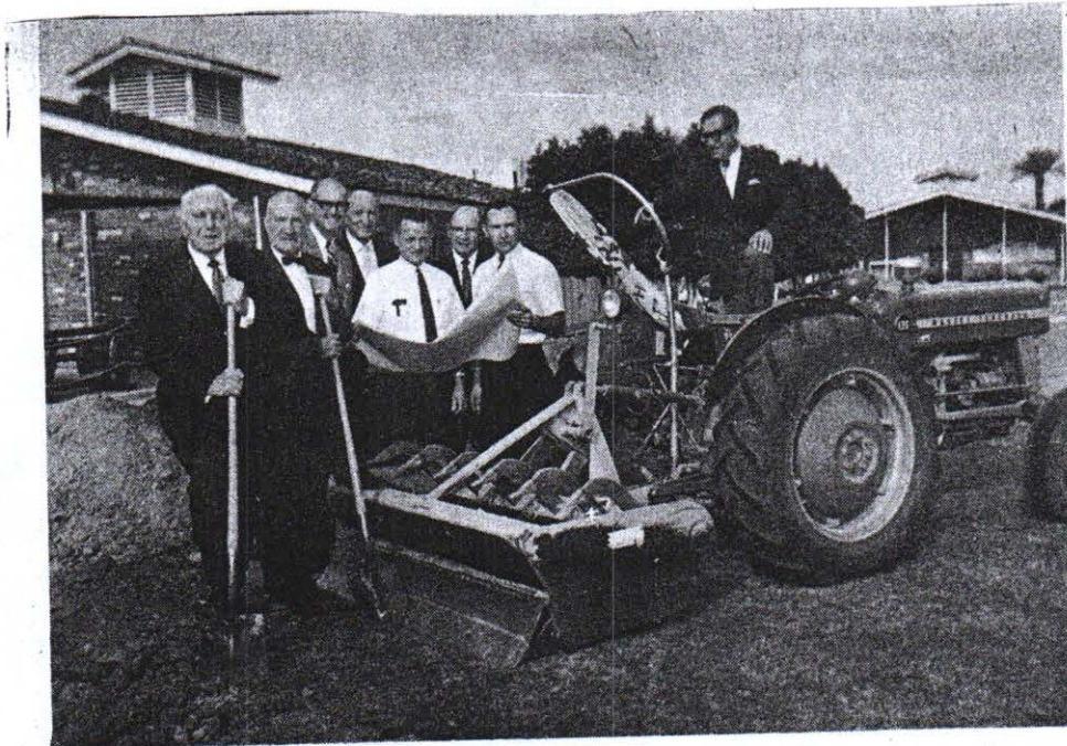
WORK STARTED — Representatives of the Sun City Community Association and Del E. Webb Development Company met last week to break ground for new shuffleboard courts as part of the Community Center
