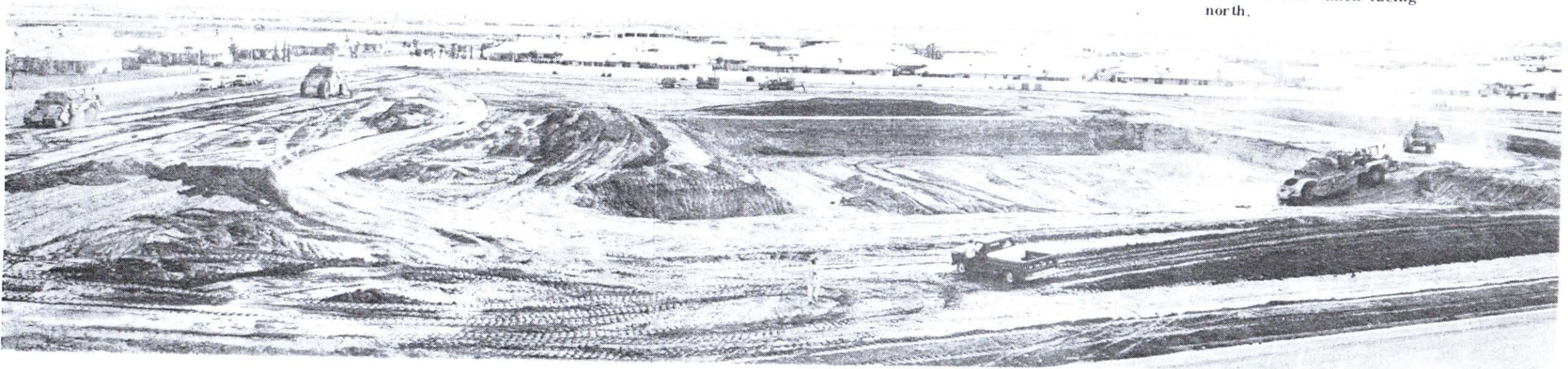
Sundial excavation began June. Photo taken facing north.
