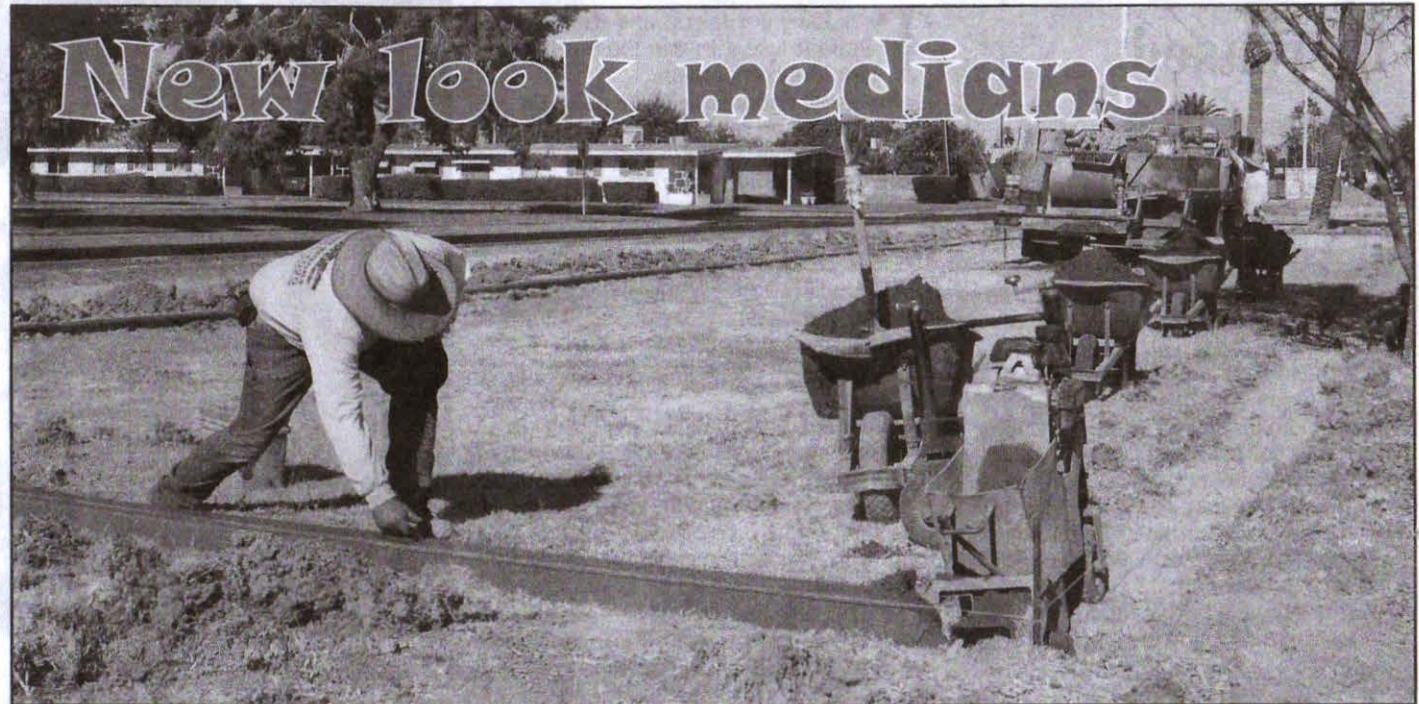
Maricopa County Department of Transportation workers install curbing in the center of medians along Peoria, Alabama and 107th avenues as part of MCDOT's renovation of the roadway areas. The new look will include grass centers with desert landscaping on the exteriors. The change will provide a more pleasing look and save on water costs.
