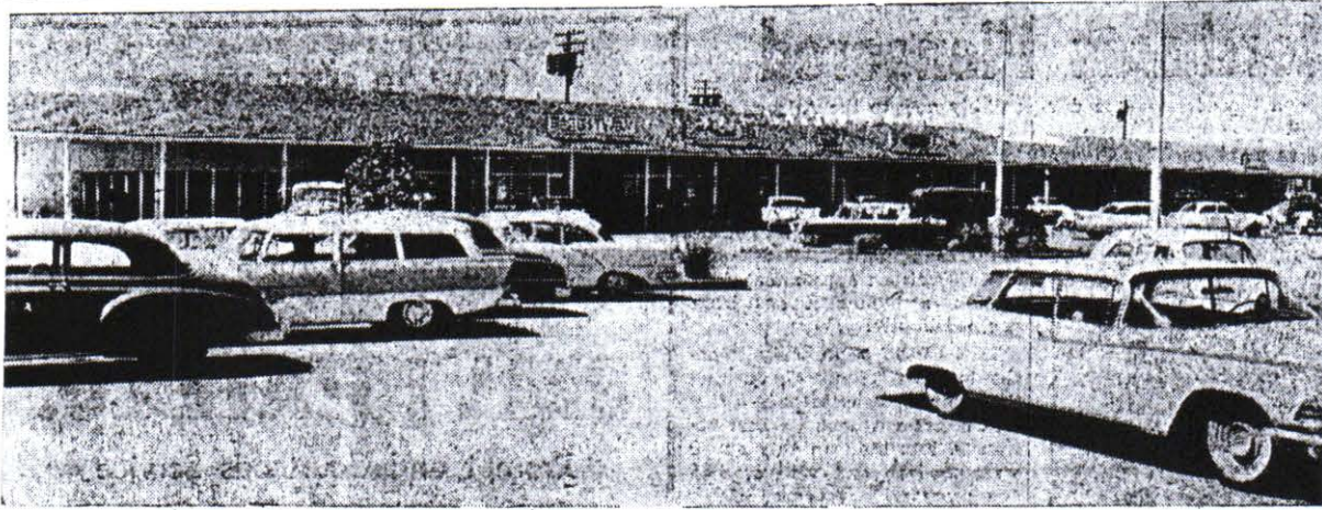
THIS IS EXPANDED Shopping Center which is nearing sta- tion as one-stop merchandise mart. Some shops are still in con- struction stage.
