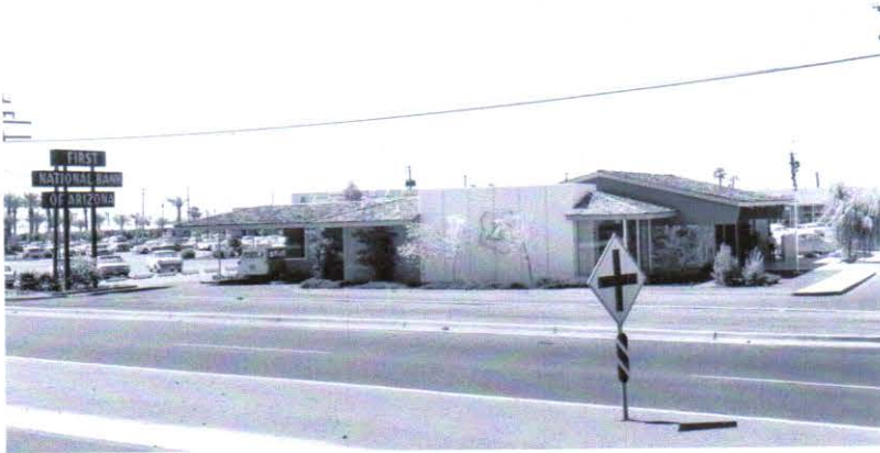
The new First National Bank of Arizona building on Grand Avenue with Grand Center in the background.
