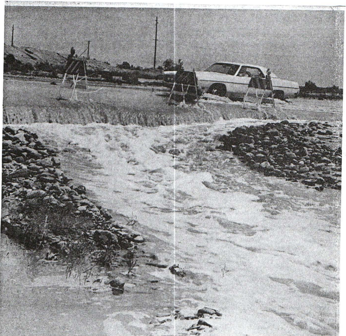
BEFORE ROAD WASHED AWAY , unidentified motorist decides to ignore warning signs and defy angry New River as it gushes over Olive Avenue following last week's heavy
