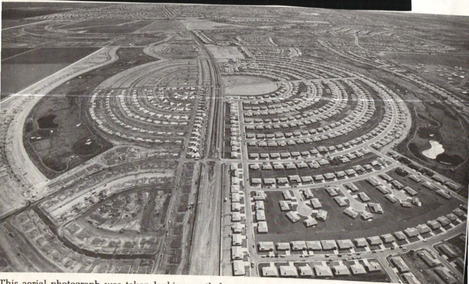
This aerial photograph was taken looking south from Sun City's northern boundary (Beardsley Road). Meandering green area at left is the new Union Hills Country Club, the community's tenth golf course. Home construction continues at fifty per week.
