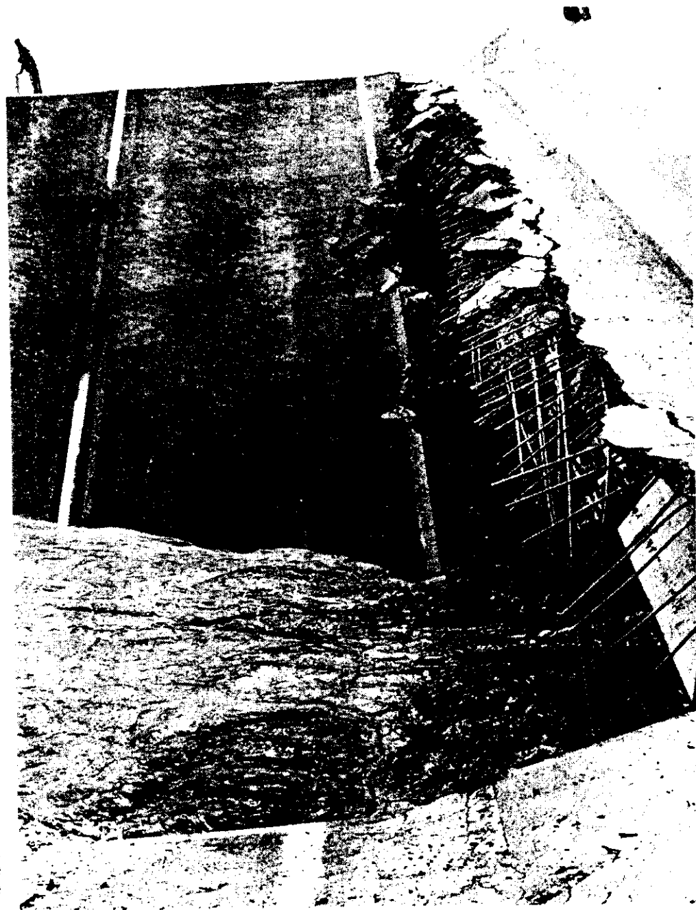
Bell Road bridge, which collapsed Friday, may not be repaired for some time, but as soon as the riverbed stops running floodwater and dries out, a temporary road will be built south and parallel to Bell Road, a county engineer says.
