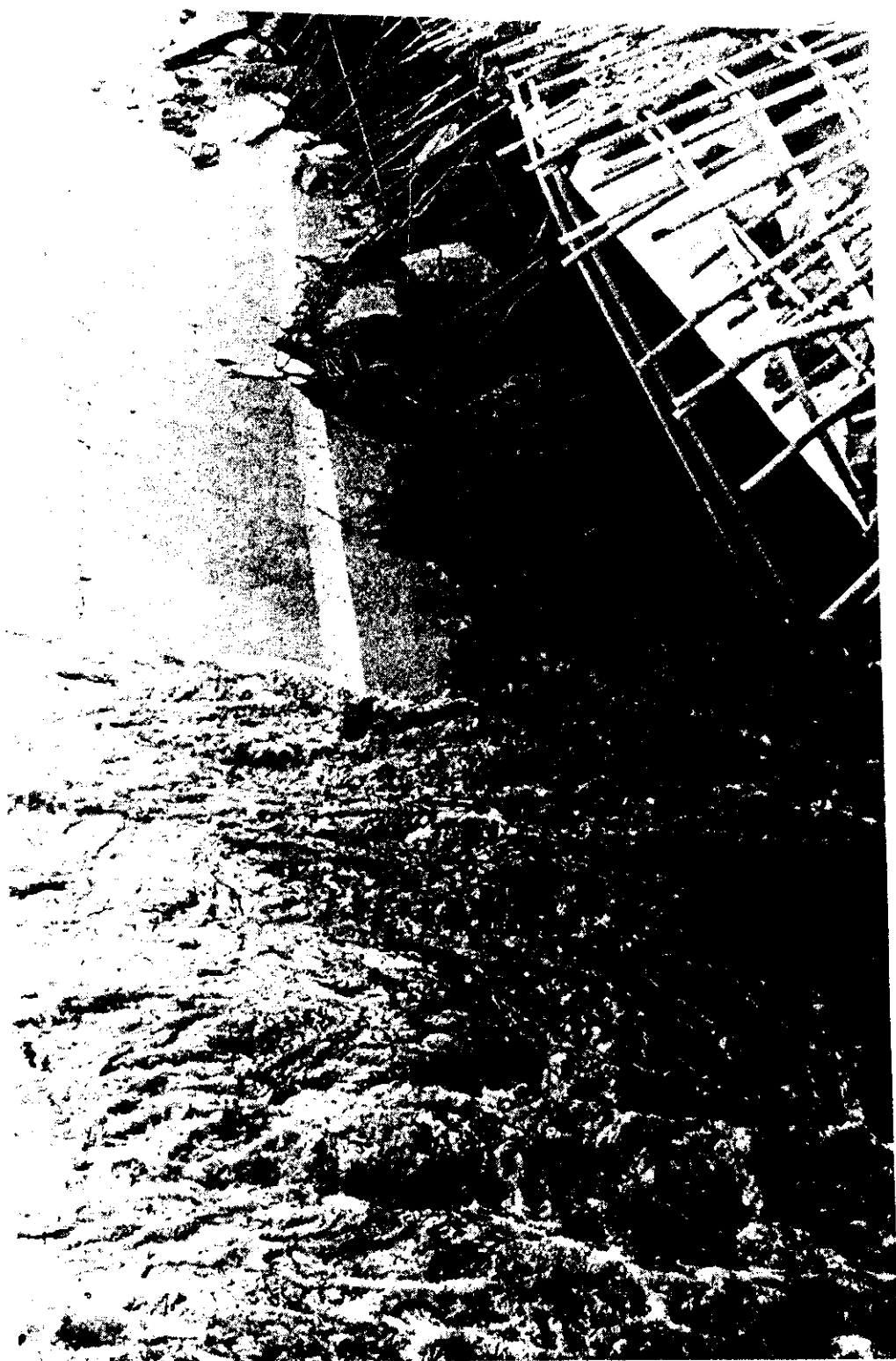
Broken by the terrible force of the water surging down the Agua Fria after release from Waddell Dam, the Bell Road bridge shows twisted steel reinforcement bars and crumbling concrete that could not hold against the river's power. As the river weakened the bridge supports, it sagged slowly until it broke.
