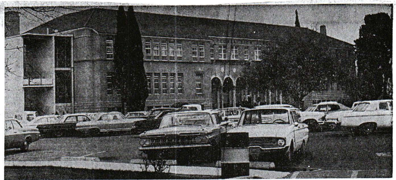
Because walls support roof, classrooms cannot be enlarged in Peoria's 1921 high school building
