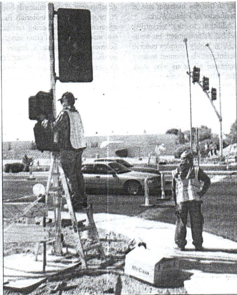
MCDOT work crews install a crosswalk sign at Aleppo and Meeker.
