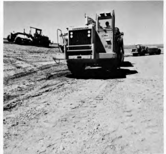
APRIL 1978 — Giant earth-moving equipment scrape and grade in what will be the core area of the community's 5,700-acre first phase.
