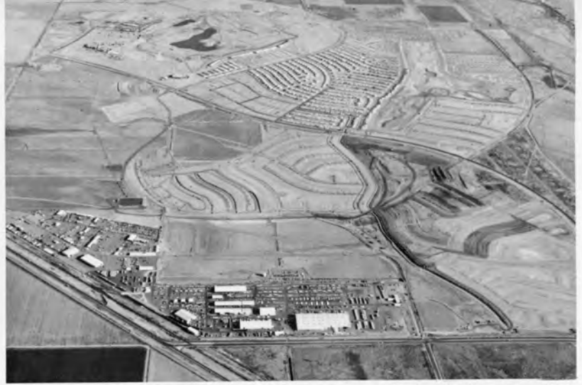
OCTOBER 1978 — As more and more homes are completed, site preparation begins for new residential sections south toward Bell Road. Water fills Hillcrest's primary lake. Bell Housing Components is at lower left.
