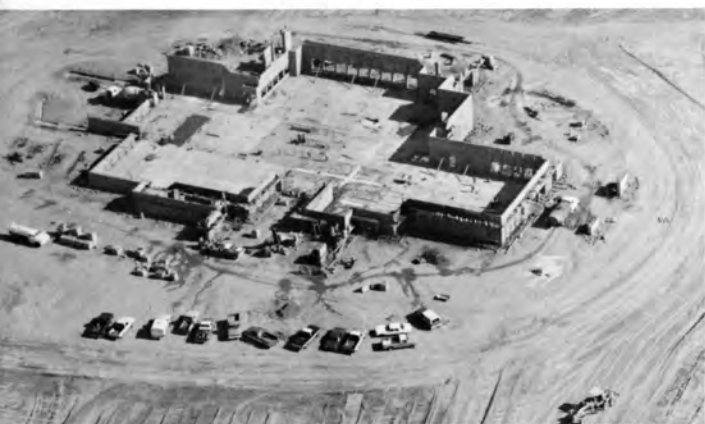
Nearly-finished walls begin to define Crestview's 30,000-square-foot facility's construction cost: $1.9 million.
