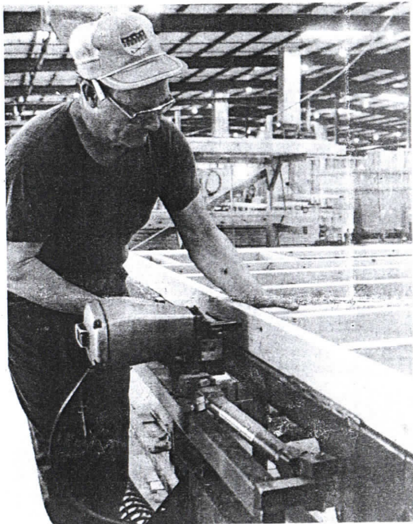
Wall panel assemblies are constructed using pre-cut members and pre-determined designs. Nailing is done with pneumatic guns.
