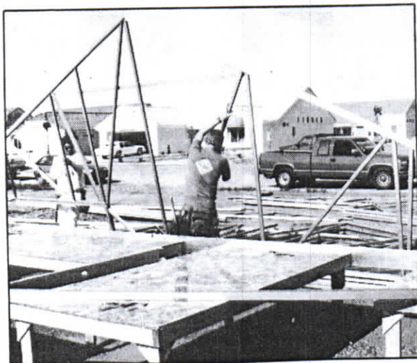
Metal trusses and studs are put in place for the new experimental SCW home.
