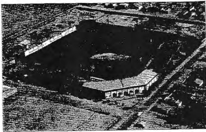
Municipal Stadium, Phoenix, where Yanks will be training.
