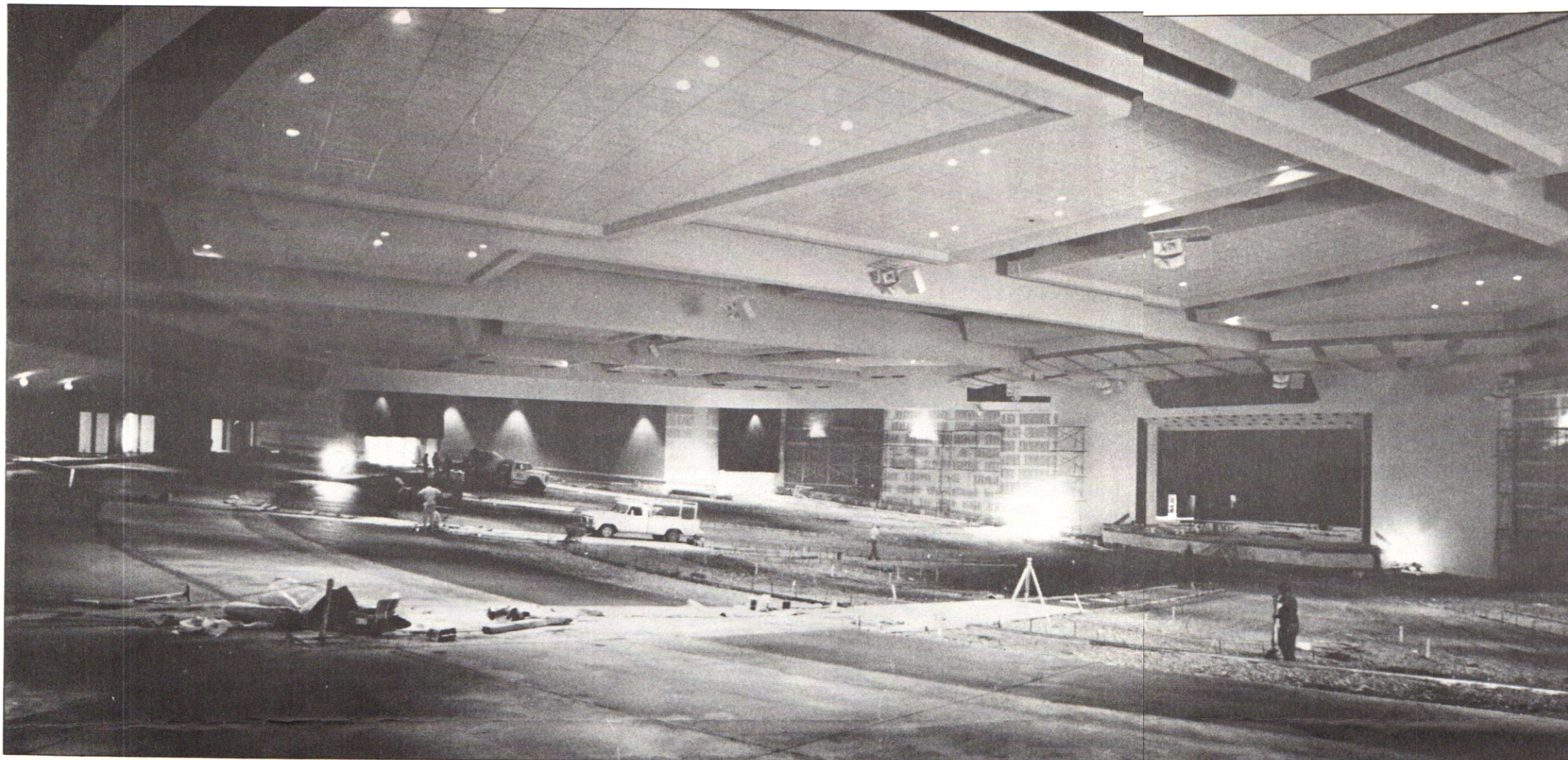
Construction crews and vehicles roam around the interior of the Sundome's main arena, diminished by its tremendous size. The theater's ramped, continental design (the floor slopes down a full 17 feet from the rear of the arena to the stage) will provide patrons
