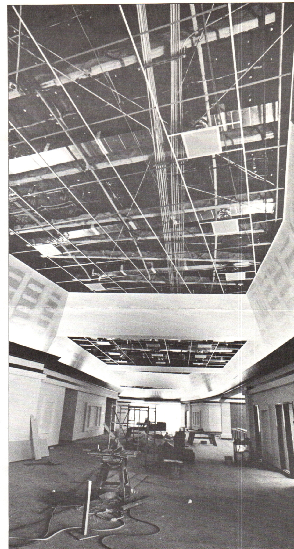
This shot of the Sundome's main entry foyer without its ceiling panels in place reveals the complexities hidden within. The trained eye can find electrical conduit, sprinkler system plumbing, roof joists, insulation, speakers and ceiling grid work. The frame-shaped projections along the foyer walls will feature photos of celebrities and movie stars. The theater also will feature a carved-stone fountain, wrought-iron gates and sparkling chandeliers, making it a true visual extravaganza.
